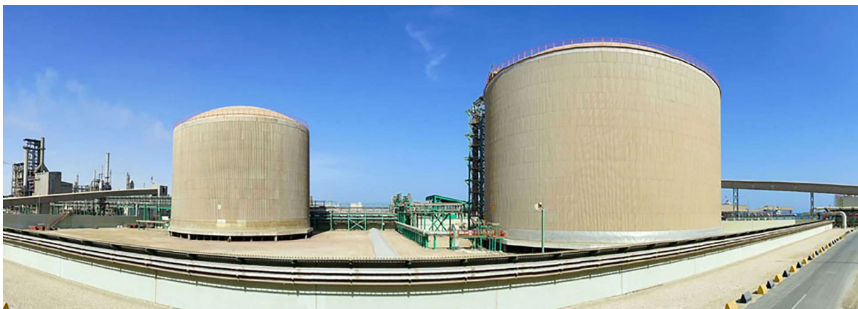
Figure 11: QAFCO's two 50,000 tonnes net capacity single-wall refrigerated ammonia storage tanks
